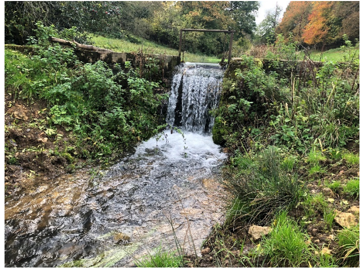
Site 5 – Man made concrete and metal barrier made impassable to migratory fish; except eel
