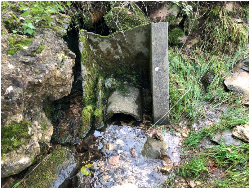
Site 4 – Pipe culvert
